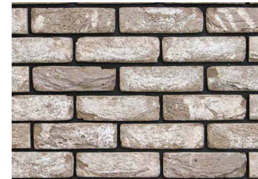
Walls - Crest Ares Facing brick walls as above
