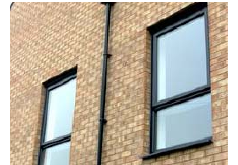
Windows Fascias - Grey uPVC with Horizontal bar style windows as above
