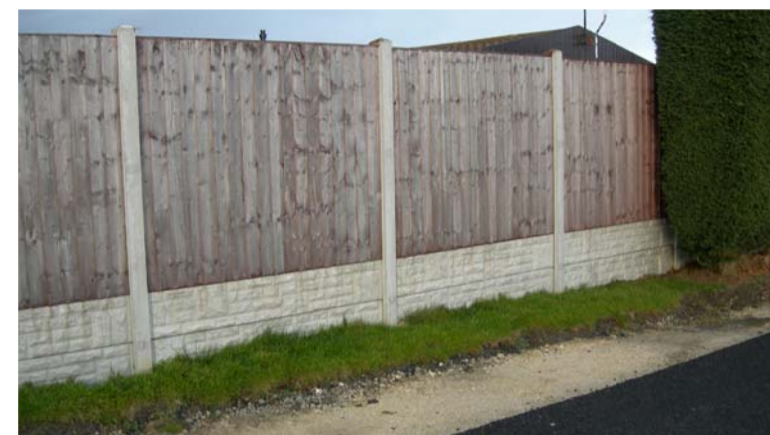
BOUNDARY TREATMENT 1 - 1.8m tall fence panels with slotted concrete posts and Gravel Boards to Eastern boundary
