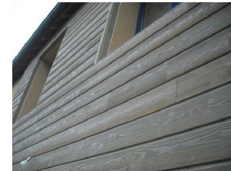
Walls - Areas of Scottish larch cladding to silver over time
